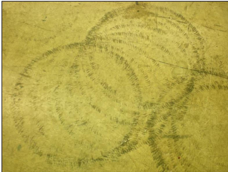
**Photo 3. Skid Steering Tracks on Concrete Floor**
